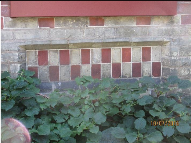
Image 6: Detail of checkerboard dichromatic brickwork detail in recessed panel.
