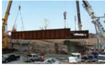
Typical Crane Positioning
