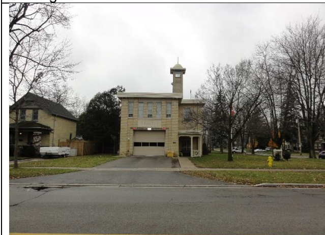
Image 11: East façade of Fire Hall No. 4. (November 25, 2016).
