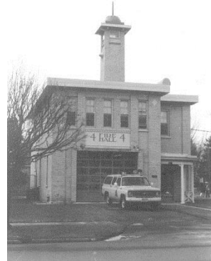
Image 2: East façade of Fire Hall No. 4, after alteration (after 1977).
