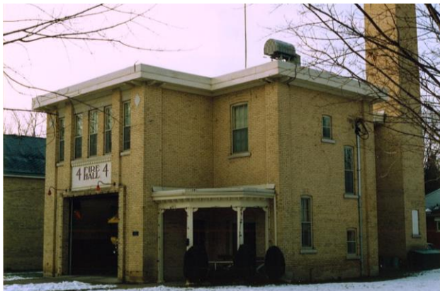
Image 3: North-east facades of Fire Hall No. 4 (c. 1986).
