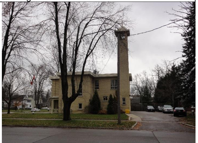
Image 12: North façade of Fire Hall No. 4 (November 25, 2016).
