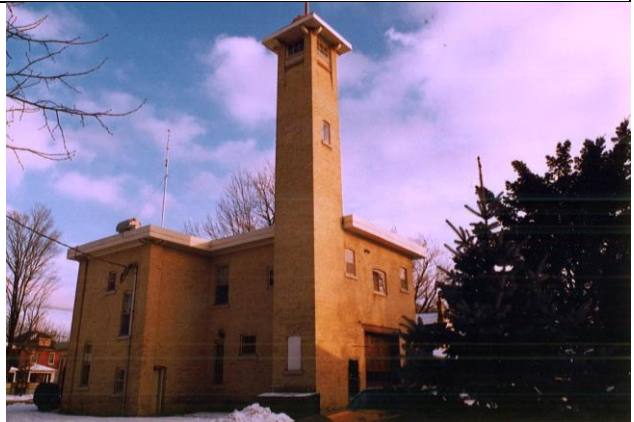
Image 4: North-west facades of Fire Hall No. 4 (c. 1986).
