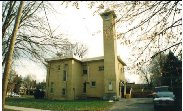
Image 6: North façade Detail of the front porch of the
