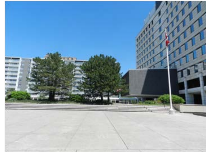
Figure 10: 532 Wellington Street (City Hall Precinct)
