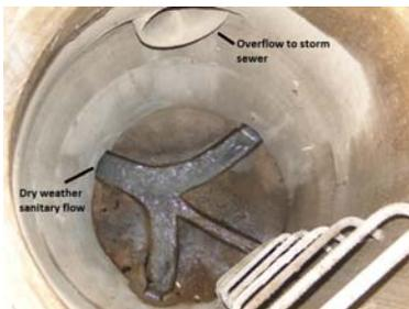
Sanitary sewer manhole with overflow to storm sewer
