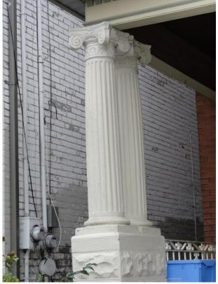
Image 4: Cast concrete column design typical on Wilkey 2½ red brick models
