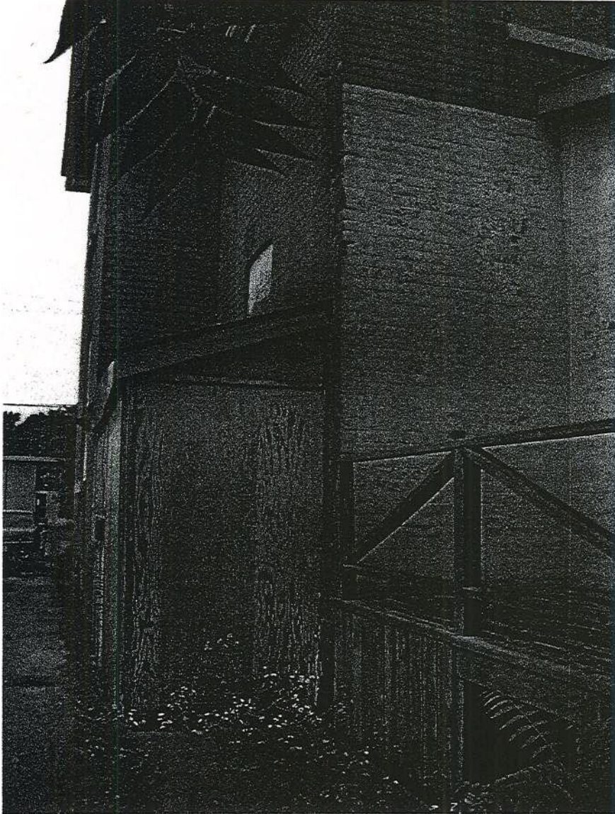
Wood enclosure over south stair accessing basement and brick damage.
