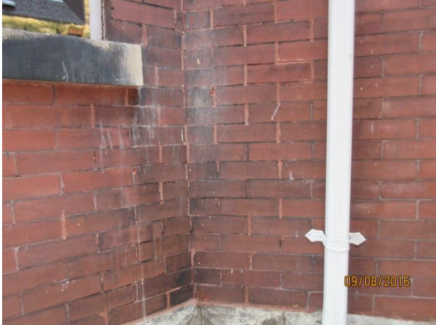
Image 9: Detail of brick showing stains (September 8, 2016).
