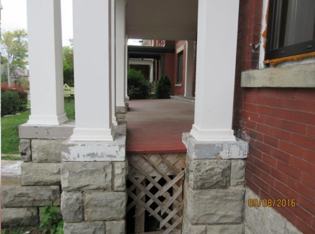
Image 8: Detail of porch piers with limestone bases (September 8, 2016).
