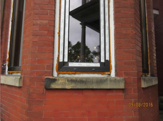
Image 10: Detail of replacement window, limestone sill, and brick (September 8, 2016).
