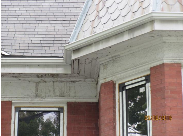
Image 7: Detail of soffit, fascia, and frieze (September 8, 2016).
