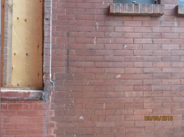
Image 12: Additional detail of brick showing stains (September 8, 2016).
