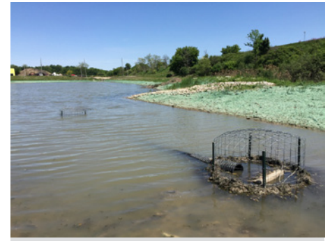
After several small rainstorms, the flow device was working well. It continued to perform just as well after a later massive storm event
