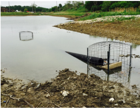
Beaver Flow Device shortly after installation
