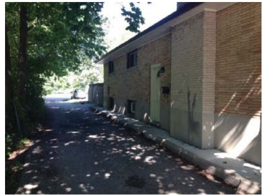
Front door of house on laneway at Raymond Street
