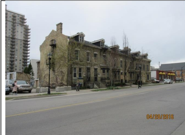
Image 1: View of Camden Terrace looking northwest.
