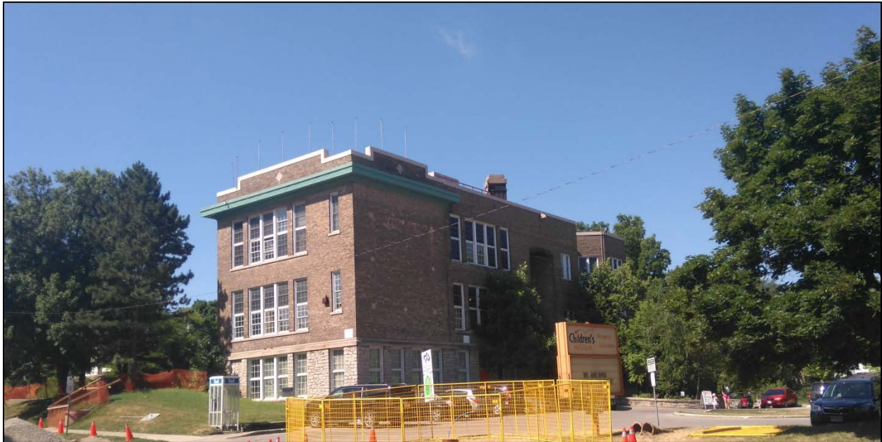
Figure 2: Existing Building Southeast Façade – July 13, 2016
