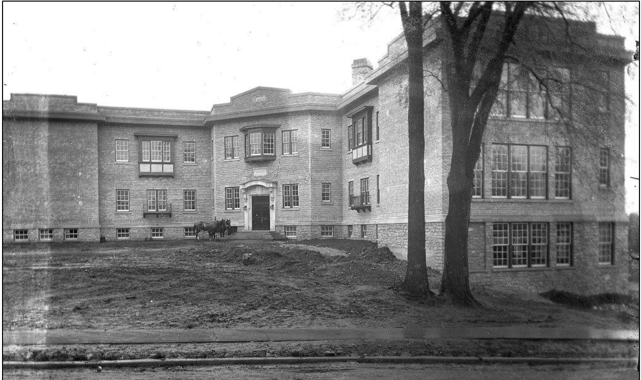
Figure 1: Riverview School Under Construction: 1916 – Courtesy of Western University: Hines Studio fonds (AFC 341-S16-117)
