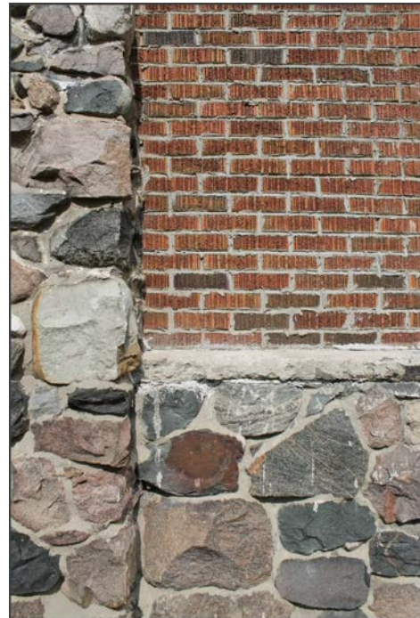
4. Split field stone plinth, concrete cap band and rug brick.
