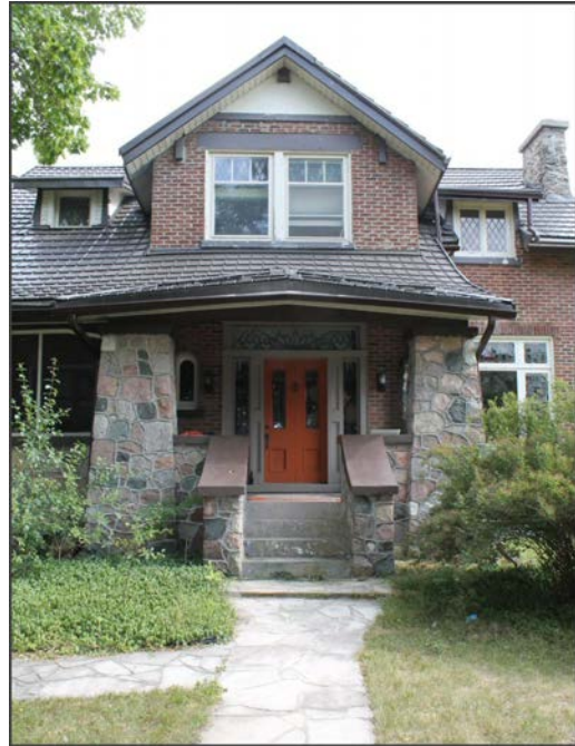
2. Front elevation of 191 Commissioners Rd
