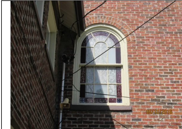
Image 9: Detail of the Georgian-style window on the east façade.
