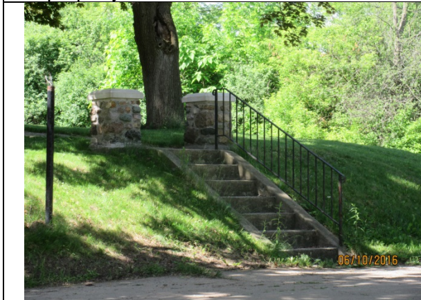
Image 3: Detail of the staircase on the front walkway.
