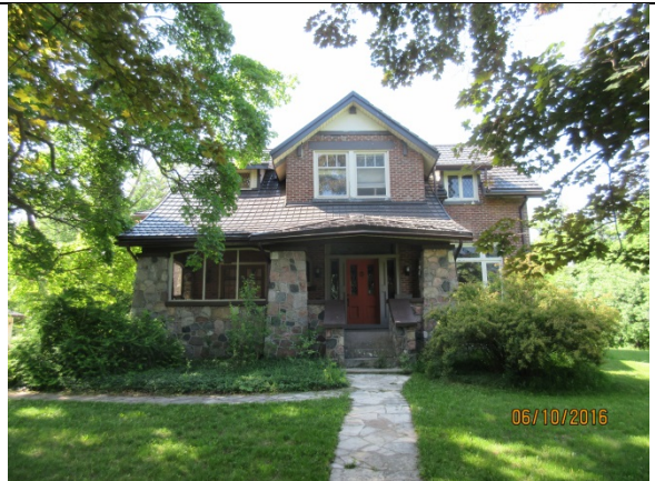
Image 4: Front (north) façade.
