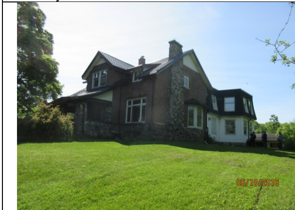
Image 5: View of north-west facades.
