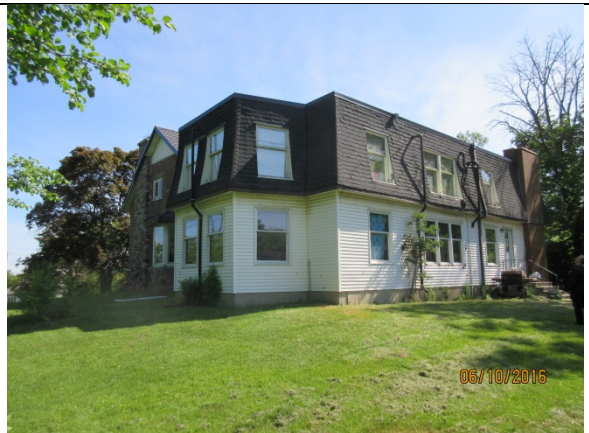
Image 6: View of south-west facades.
