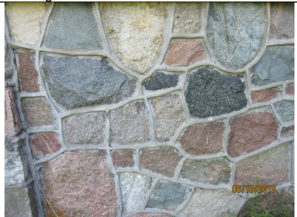
Image 14: Detail of the fieldstone with raised joints.
