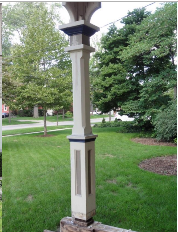
Image 3: Front (south) detail of existing west column being replaced
