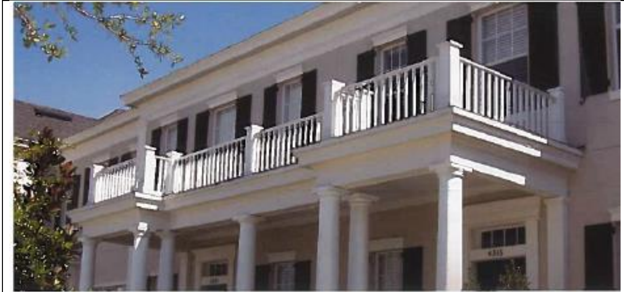
Image 7: Azek synthetic material used for porch trim and column surrounds
