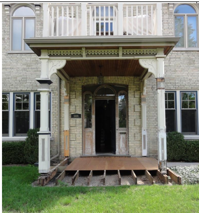
Image 2: Front façade, detail of porch during tear-back
