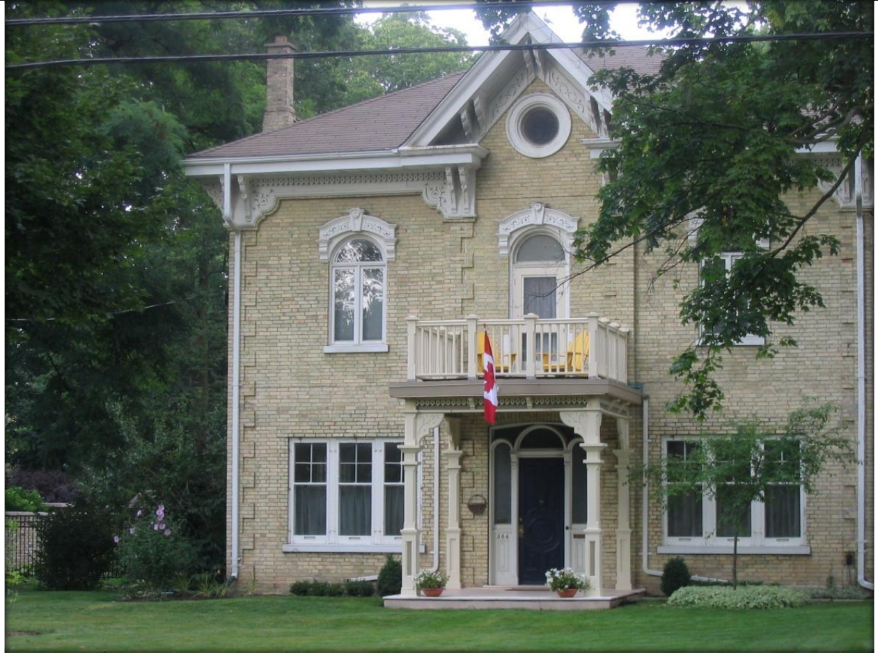
Image 1: Front façade, south, of the building
