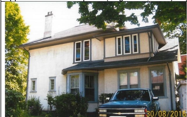
Image 9: West façade (B. McDougal).
