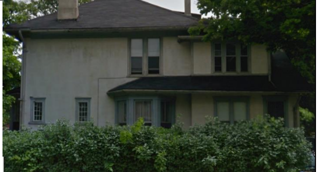
Image 2: West façade of building at 183 Bruce Street prior to window replacement.
