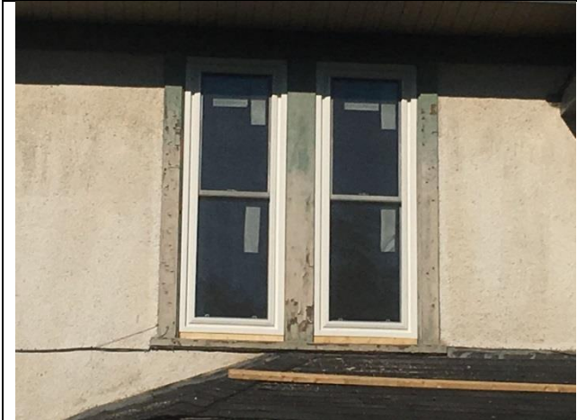
Image 5: Detail of replacement window on upper front façade (August 10, 2016).
