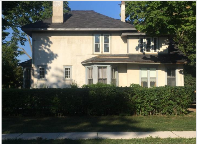
Image 4: West façade of building at 183 Bruce Street after window replacement (August 10, 2016).
