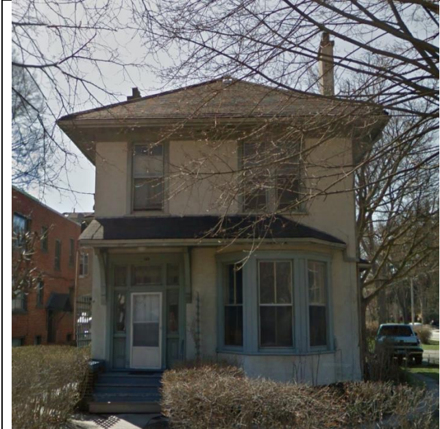
Image 1: Front façade (north) of building at 183 Bruce Street prior to window replacement.
