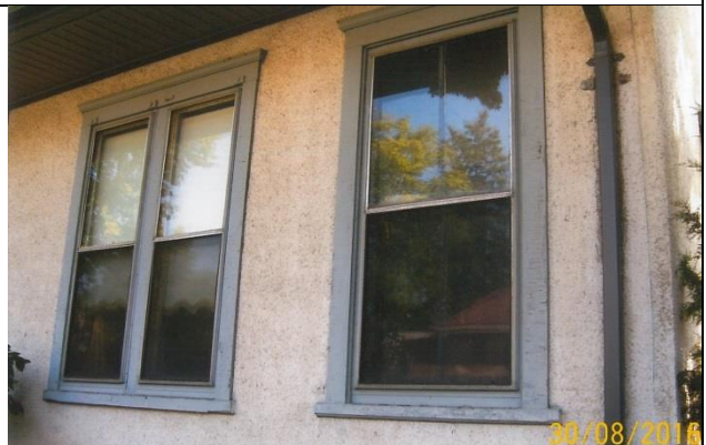
Image 10: Detail of windows and trim (B. McDougal).
