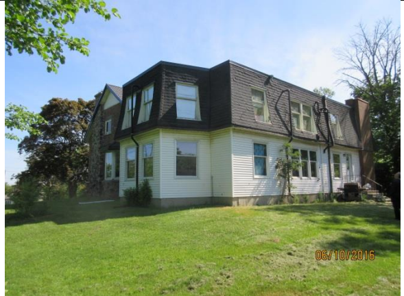
Image 6: View of south-west facades.
