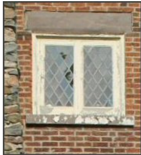
9. Harlequin pattern leaded glass casement window. This was popular with the Tudor Revival style within the Arts and Crafts Movement.
