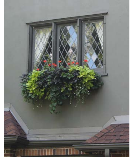
25. An example of a harlequin pattern leaded windows on Base Line Road. The use of leaded glass is not uncommon in Old South London north of Commissioners Road. A successful London hardware store, Hobbs Hardware, at one time employed 9 decorative glass glazers in their London workshop.
