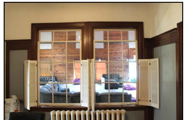
15. Formerly exterior windows of the hearth room now open onto the former enclosed pool.
