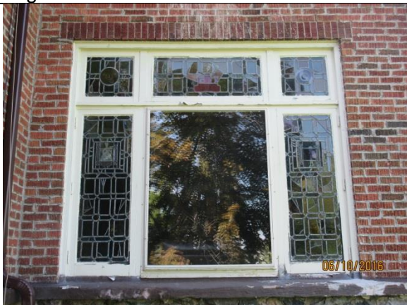
Image 7: Detail of the front ledged window.
