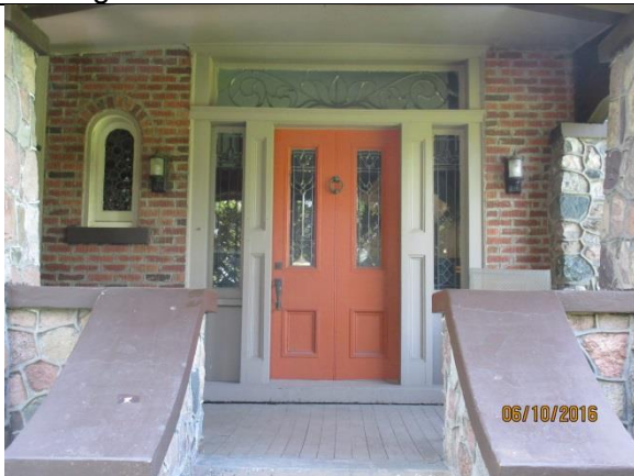
Image 13: Detail of the front door.
