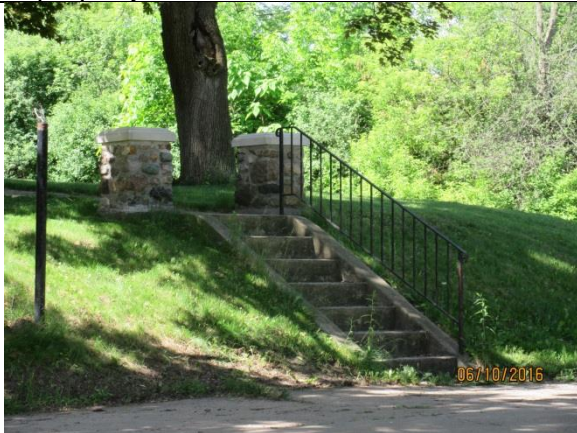
Image 3: Detail of the staircase on the front walkway.
