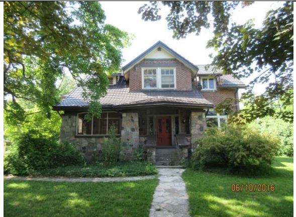
Image 4: Front (north) façade.
