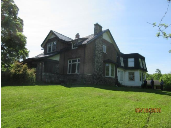
Image 5: View of north-west facades.
