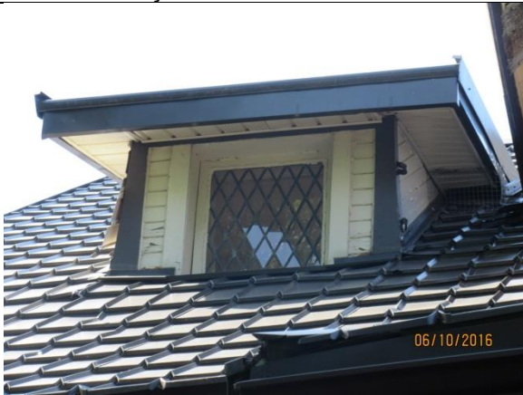
Image 11: Detail of the shed dormer with leaded glass window.
