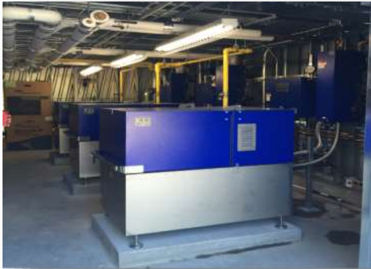
New Combined heat and Power System
