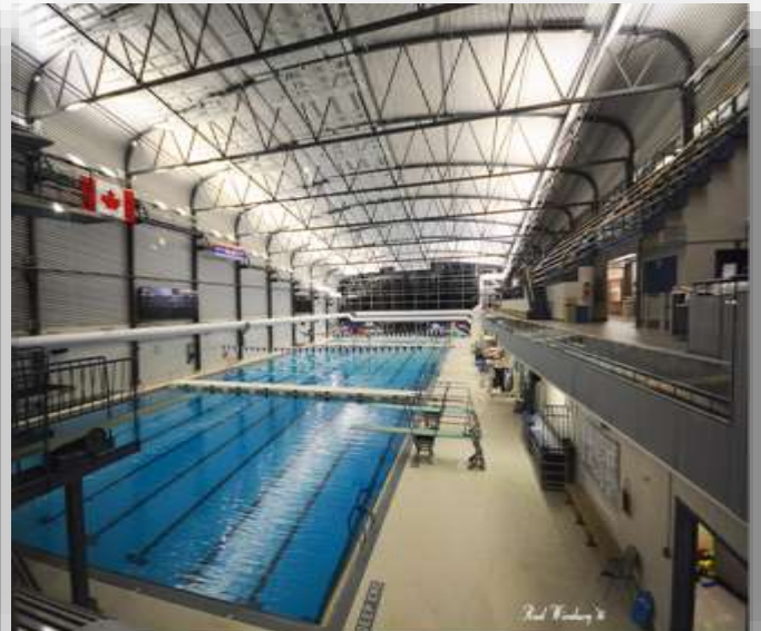
Pool area building with new lighting, bulkheads, acoustic treatments
