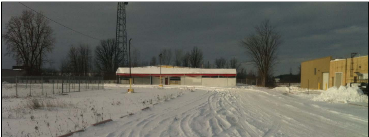
Figure 1: Existing Building (Site visit Jan, 2016)
