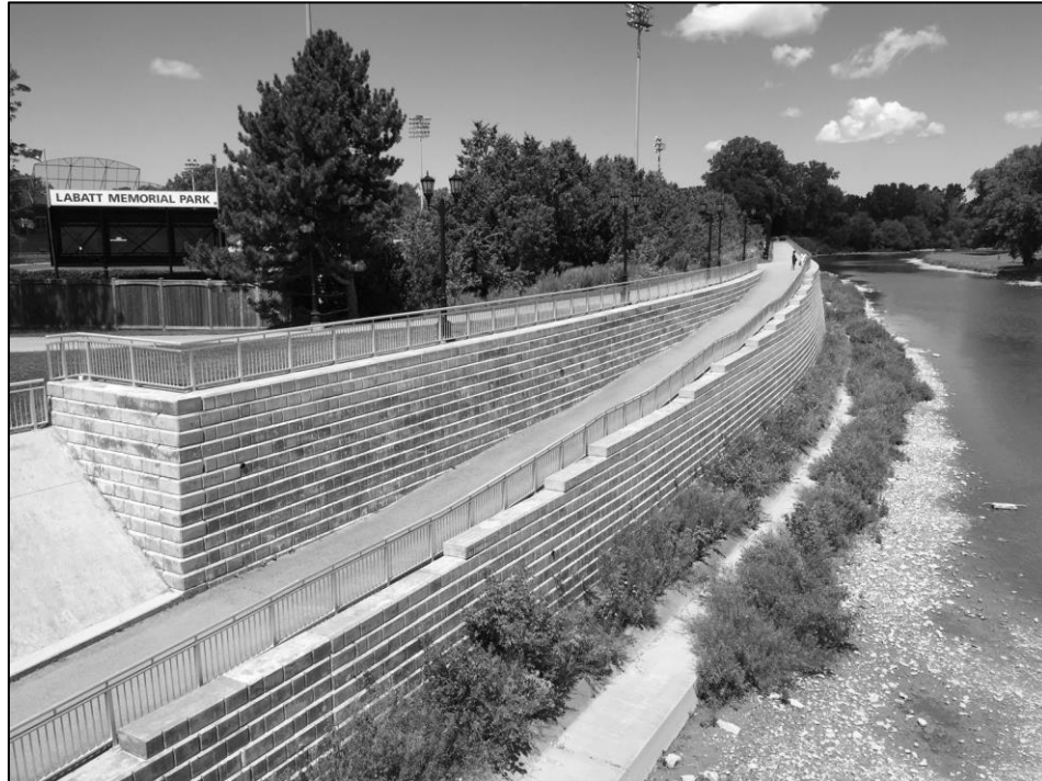
Figure 1 Phase 1 of West London Dyke Replacement.
