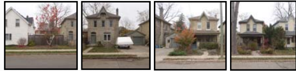
64 72 Subject lands 66 68 70 North side view
