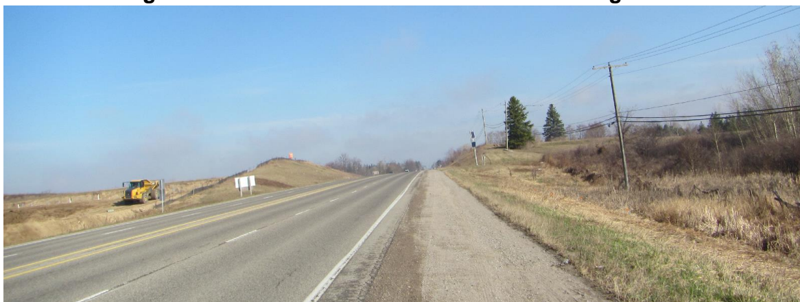
Figure 1: Site Photo – Richmond Street Looking North
