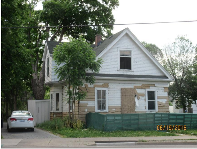
Image 1: Main (east) façade of 102 Wharncliffe Road North.
