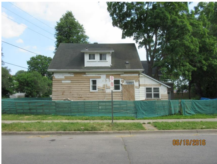
Image 2: North façade of 102 Wharncliffe Road North.
