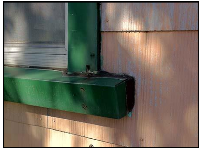
Figure 10. Exterior window surround
