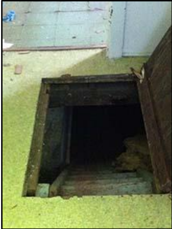
Figure 8. Trap door to basement and crawl space
