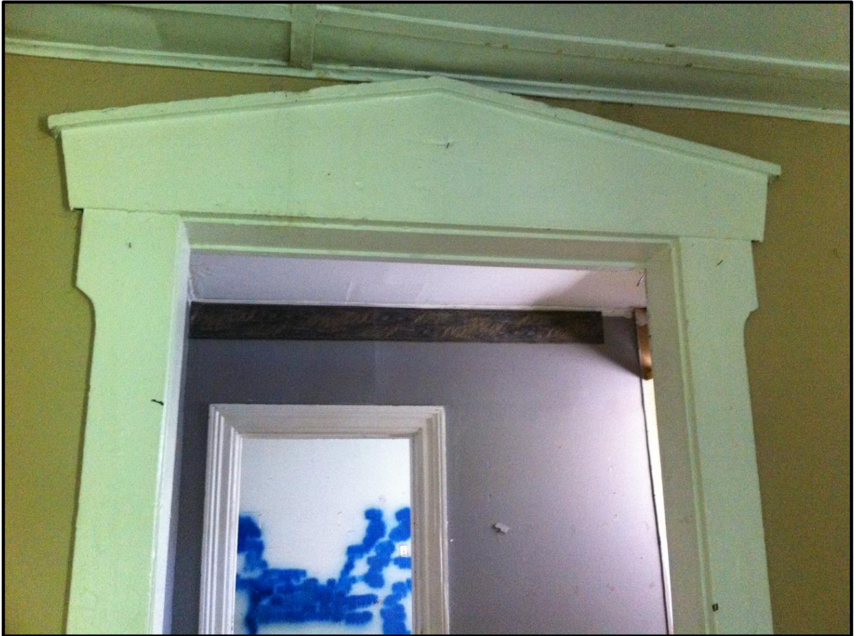
Figure 13. Interior door surround resembling Fugitive Slave Chapel exterior window trim profile
