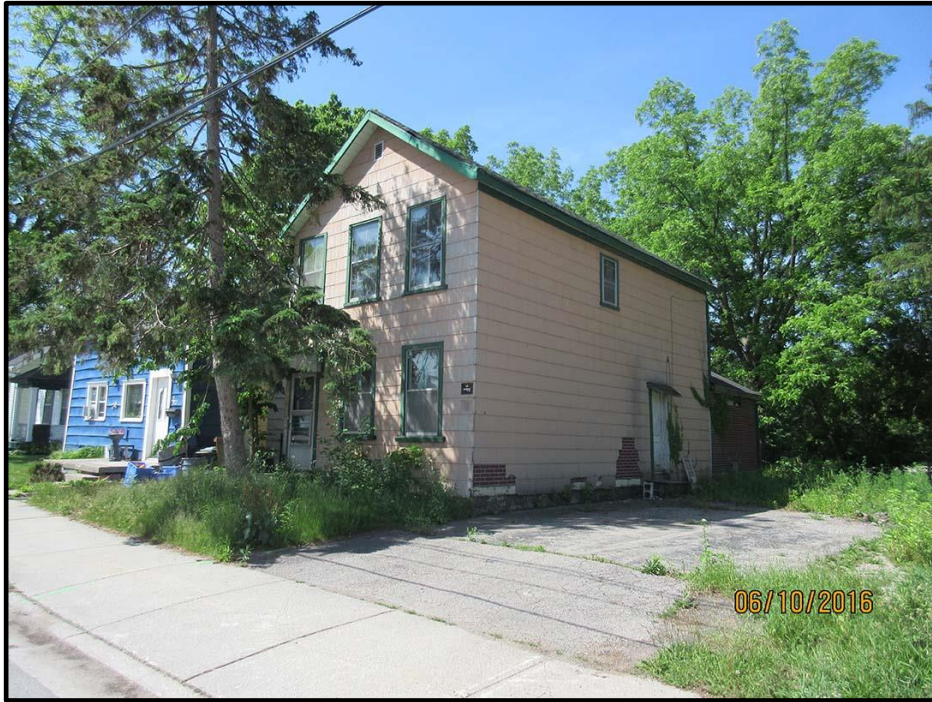
Figure 5. Front-corner of 269 Thames Street
