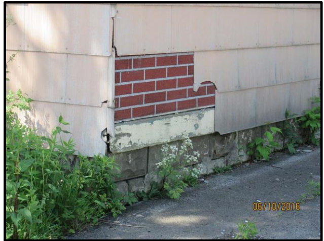
Figure 9. Construction of exterior wall and foundation
