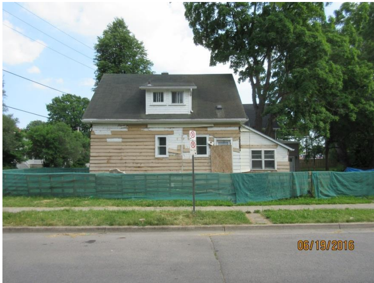
Image 2: North façade of 102 Wharncliffe Road North.
