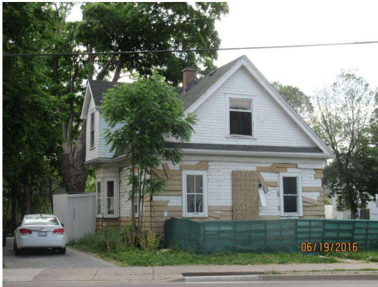
Image 1: Main (east) façade of 102 Wharncliffe Road North.
