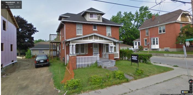
Image 1: 216 Wharncliffe Road North (July 2009, courtesy Google).
