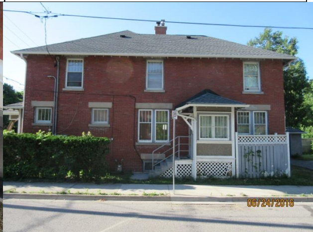
Image 8: North façade of the building located at 216 Wharncliffe Road North.
