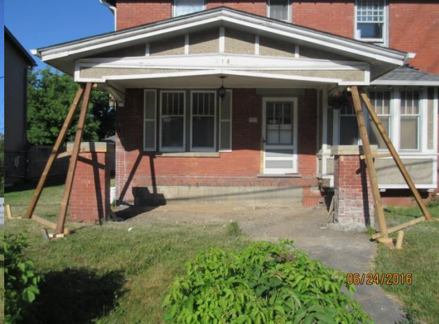
Image 4: Detail of porch on the building at 216 Wharncliffe Road North.
