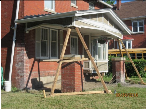
Image 5: Detail of porch on the building at 216 Wharncliffe Road North.
