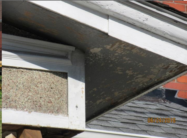
Image 6: Detail of the sloping soffit of the porch.
