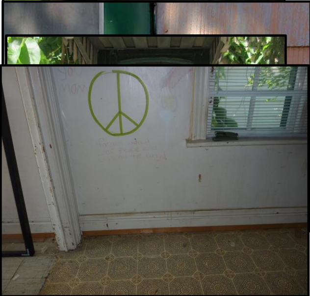
Figure 8. Trap door to basement and crawl space
