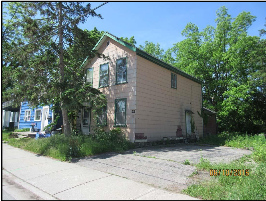
Figure 5. Front-corner of 269 Thames Street
