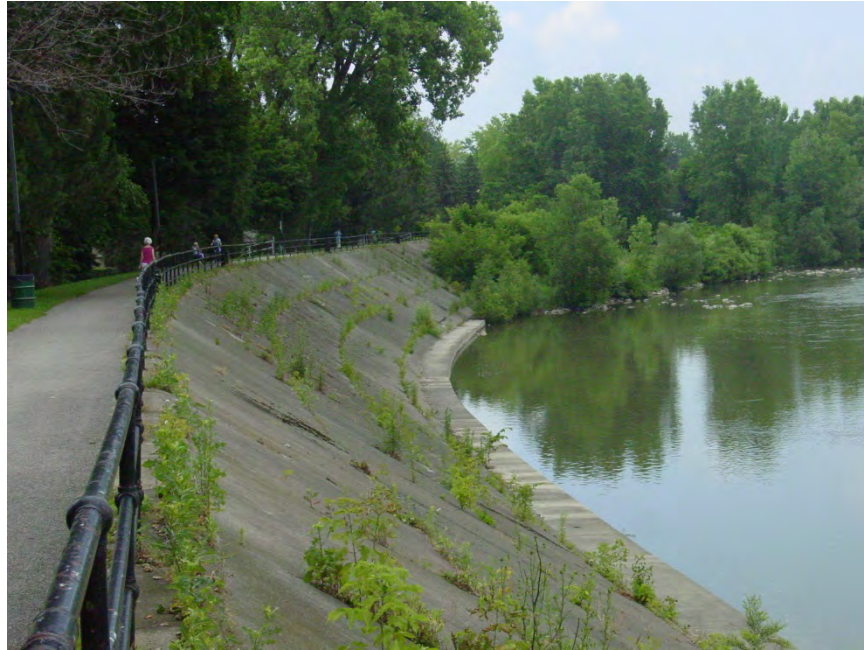
Plate 3: View of the West London Dyke and greenway looking north
