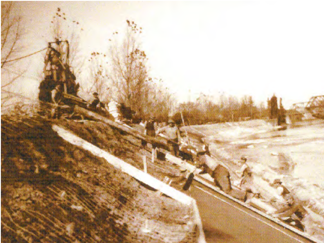
Plate 1: Concrete facing of the West London Dyke c.1930s
