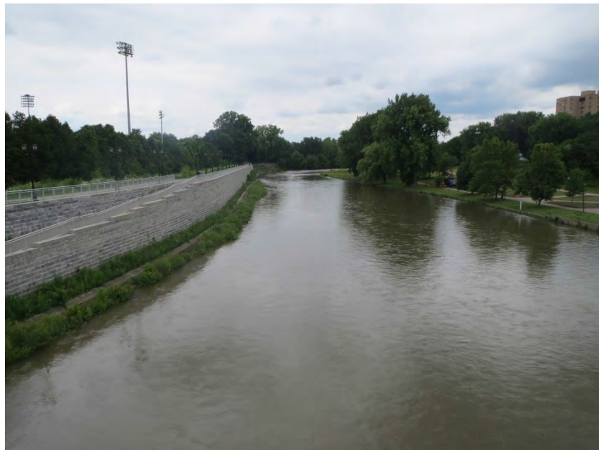
Plate 4: View looking north of the section of the Dyke rebuilt in 2007 (adjacent to Labatt Park)
