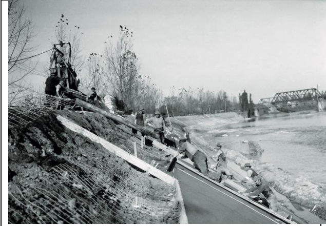
Image 1: Slope protection along the West London Dyke (prior to 1937).
