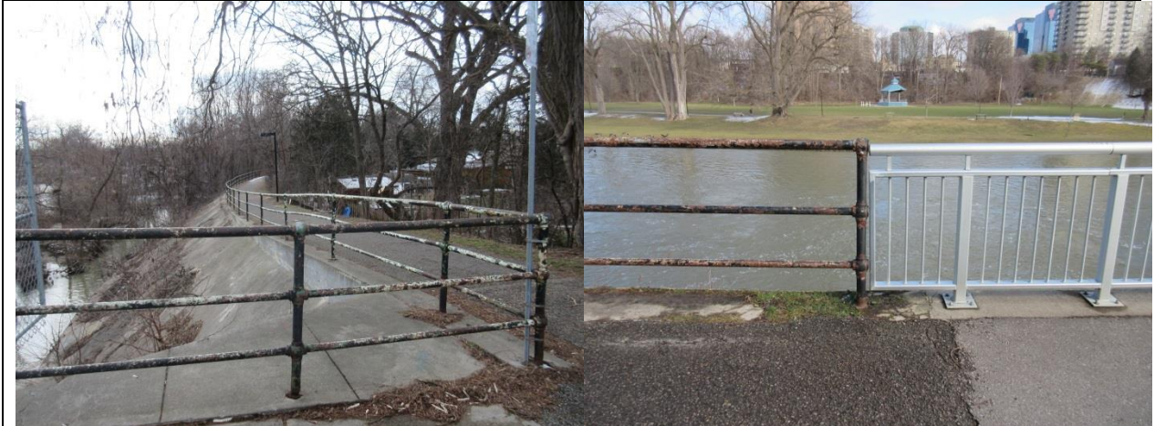
Image 7: Detail of historic railing along West London Dyke, near Blackfriars Bridge.
