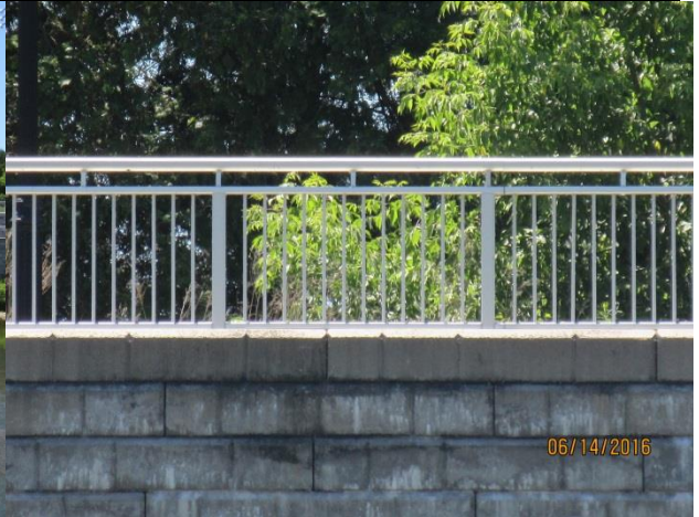
Image 4: Detail of railing replaced in 2007.
