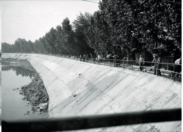
Image 2: Slope protection along the West London Dyke; work completed (prior to 1937).
