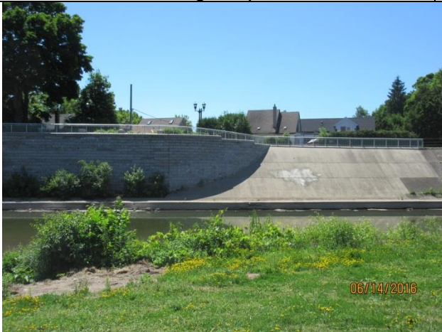
Image 5: Junction of new and historic dyke near Rogers Avenue, seen from Harris Park.
