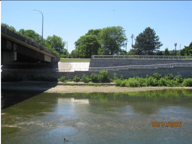
Image 3: West London Dyke adjacent to Queens Avenue Bridge, replaced in 2007.
