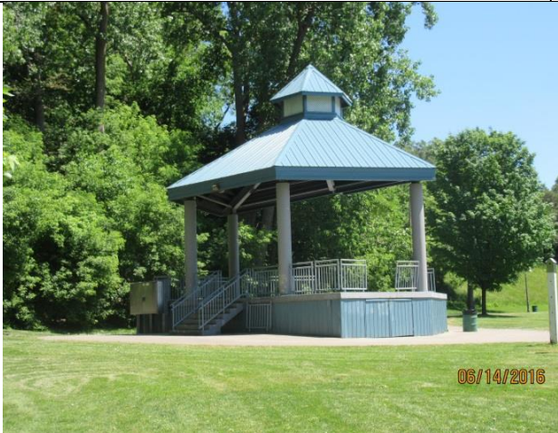
Image 3: Harris Park pavilion, rear (north) view.
