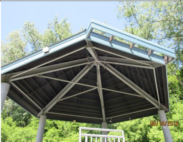
Image 5: Detail of the roof structure of the Harris Park pavilion.
