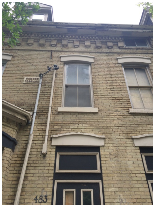
Plate 4 Brick work and wide eaves
