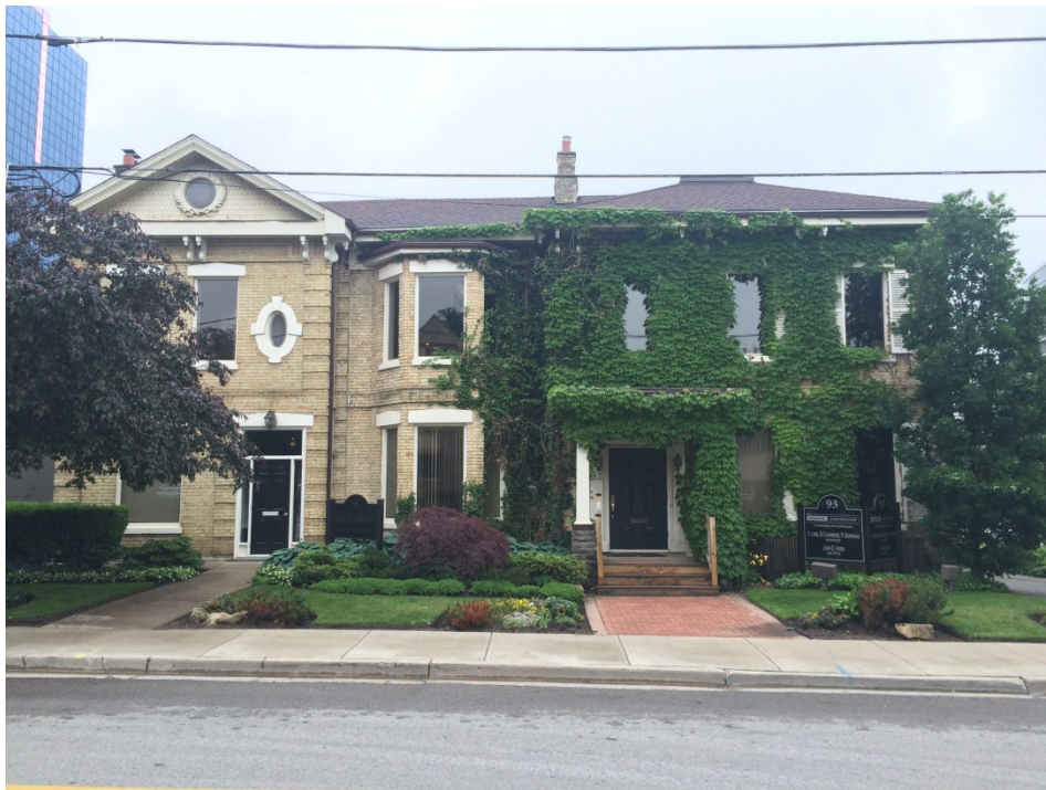
Plate 7 Front facade, or south view, 93/95 Dufferin Avenue
