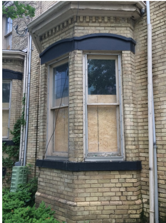
Plate 3 Bay window, 483 Talbot Street
