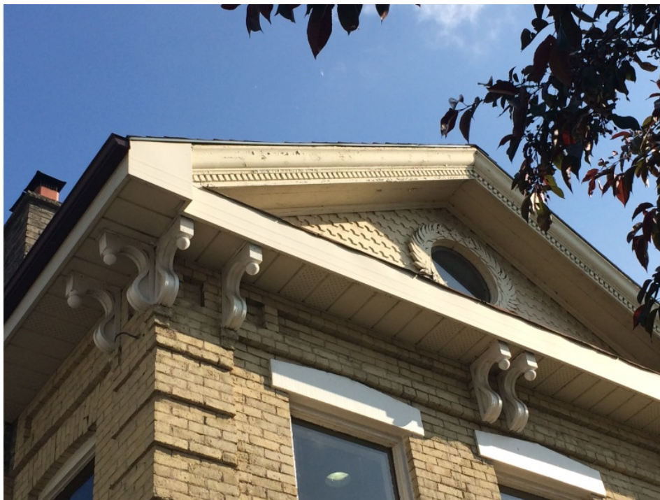
Plate 10: Eaves, cornices and pediment at 95 Dufferin Avenue
