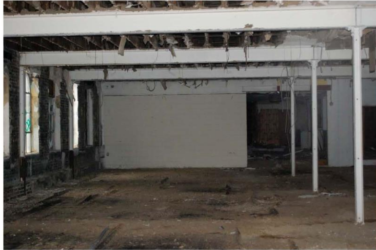
Photograph 35: Hollow Concrete block wall at the second floor level.
