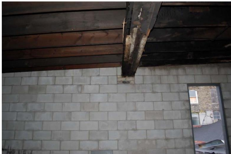
Photograph 34: North wall of south addition from the interior.
