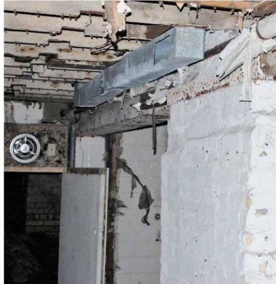
Photograph 12: Access door (lower left) to south crawlspace with pier beyond.
