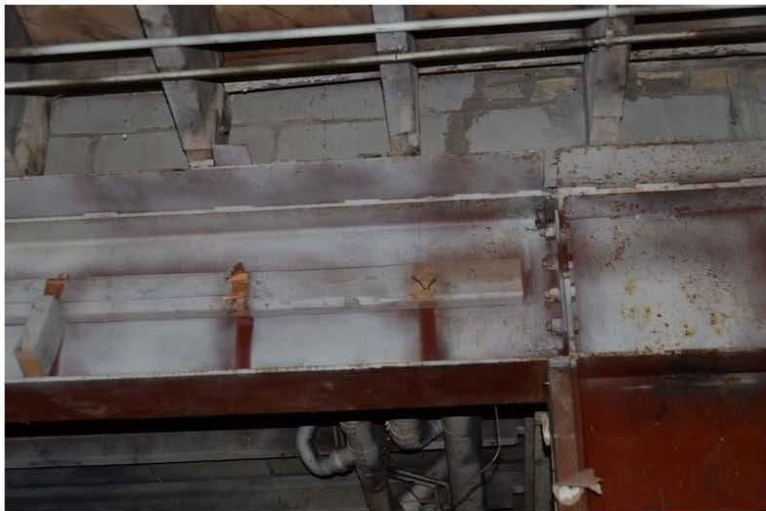
Photo No. 11: Rigid Frame Supporting Masonry Wall
