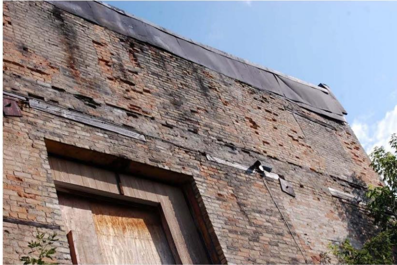
Photograph 31: South wall, third floor at the east end.
