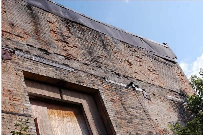
Photograph 24: South wall, third floor at the east end.
