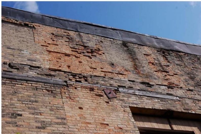
Photograph 30: South wall, third floor at the midpoint.
