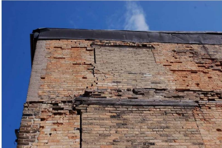
Photograph 29: South wall, third floor at the west end.
