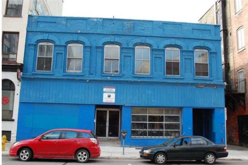
Photograph 1: North elevation fronting on King Street.
