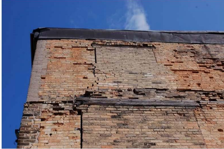
Photograph 22: South wall, third floor at the west end.
