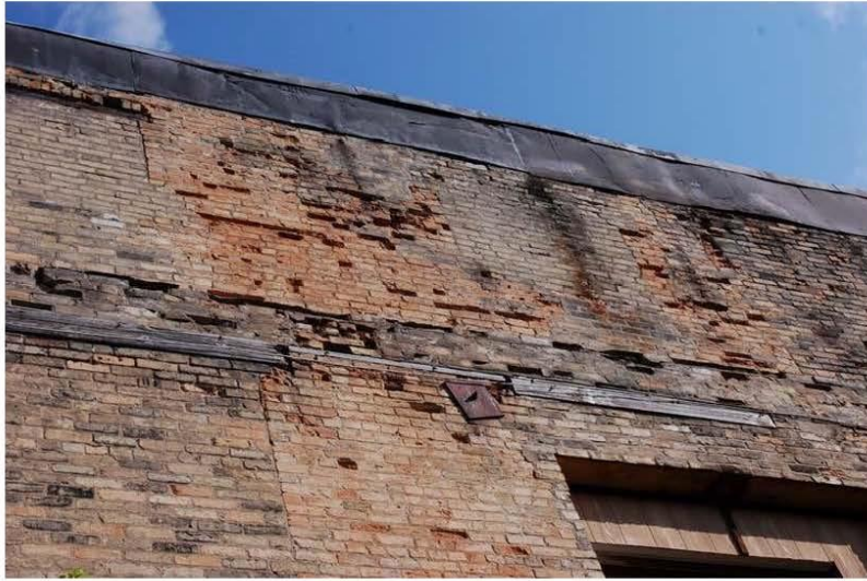
Photograph 23: South wall, third floor at the midpoint.
