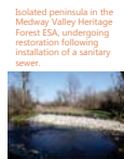
Isolated peninsula in the Meadow Valley Heritage Forest ESA, undergoing restoration following installation of a sanitary sewer.
