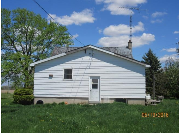
Image 3: Rear (west) façade of the house located at 5221 Cook Road.
