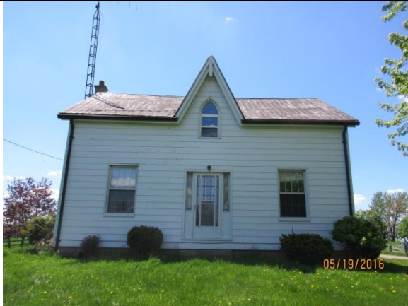
Image 1: The front (east) façade of the house located at 5221 Cook Road.
