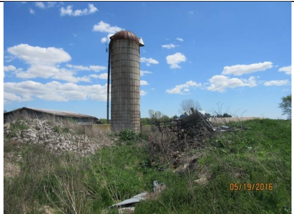
Image 6: Former barn with standing silo at 5221 Cook Road.
