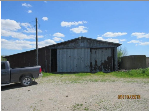
Image 5: Drive shed located at 5221 Cook Road.
