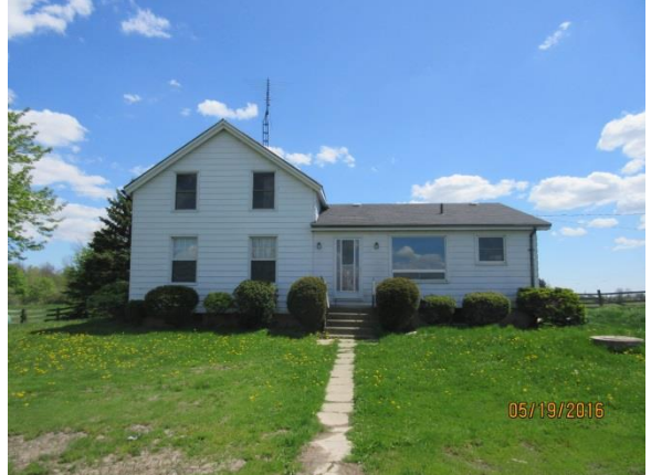
Image 4: North façade of the house located at 5221 Cook Road.
