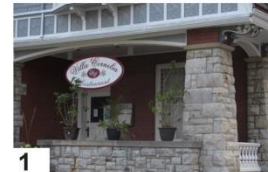
1 Richardsonian Romanesque stone block foundation, verandah railing and support
