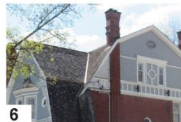
6 Shingle clad cross gambrel roof
