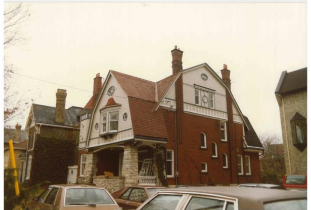
Image 7: Restoration work complete (c.1989).
