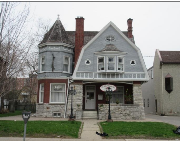
Image 12: Front façade (April 30, 2015).
