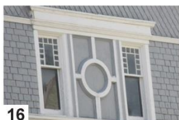
16 Detail of upper east elevation paired window with decorative panel
