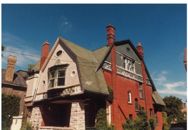
Image 6: Restoration work underway (c.1988).
