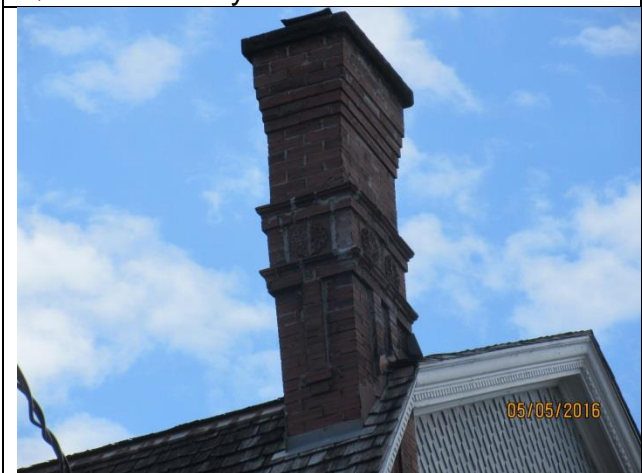
Image 19: One of the three chimneys.
