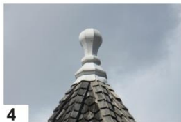
4 Conical roof and finial of turret
