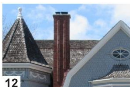
12 Tall, elaborate brick chimney
