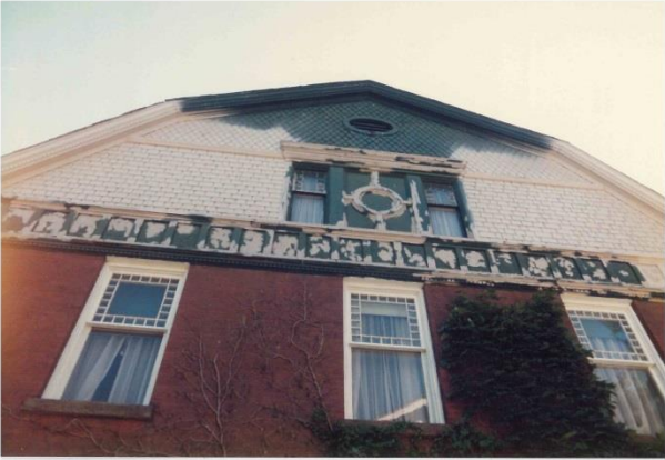
Image 6: Detail of restoration work on west façade (c.1988).
