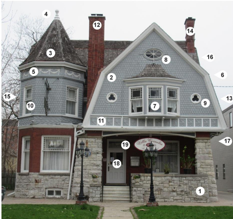
1 Richardsonian Romanesque stone block foundation, verandah railing and support
