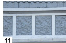
11 Square, rusticated, tin panels
