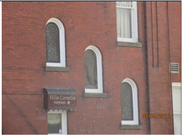
Image 14: Ascending windows on the staircase, east façade.
