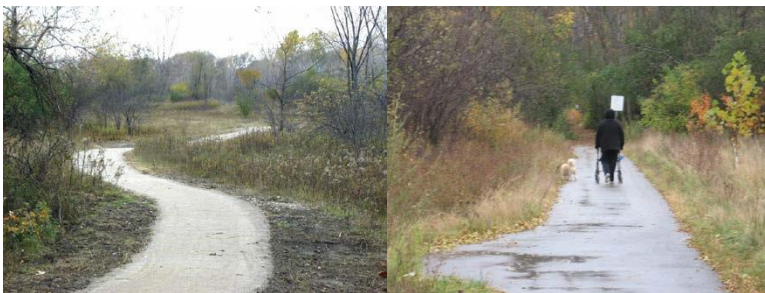
Two types of Level 2 Trails. On the far left is a limestone screening trail through an old field / savannah habitat in Killaly Meadows ESA. On the right is a paved trail overlying a sanitary sewer maintenance access in Westminster Ponds ESA.
