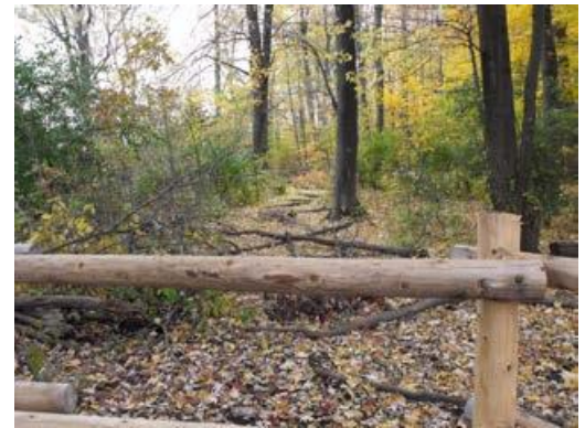
Cedar post and rail barricade and logs placed on the closed trail segment at Forest View Heritage Woodland Park.
