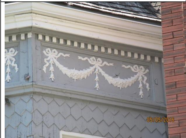
Image 15: Swag and garland detail on the cornice frieze of the turret.
