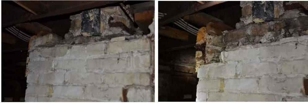
Photo No. 05 & 06: Crumbling Masonry Pier
