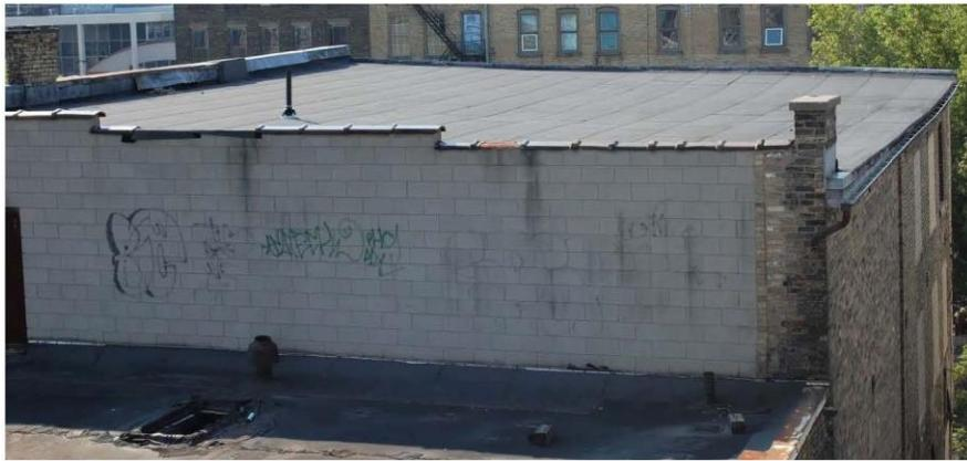
*Photograph 33:* North wall of south addition. Hollow concrete block capped with clay tile capping.
