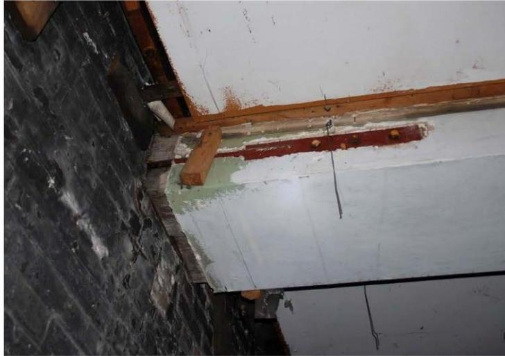
*Photograph 41:* Rod assembly with exterior wall plate to restrain the masonry wall.
