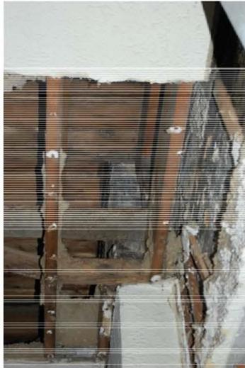
*Photograph 44:* Approximately 1" +/- movement of sheathing away from wall. No positive connection between roof framing and masonry.
