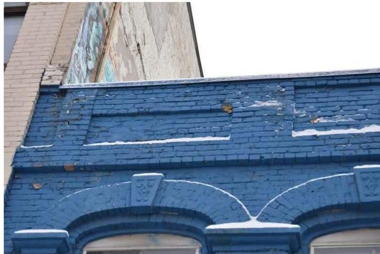
Photo No. 02: Delaminating Masonry Parapet
