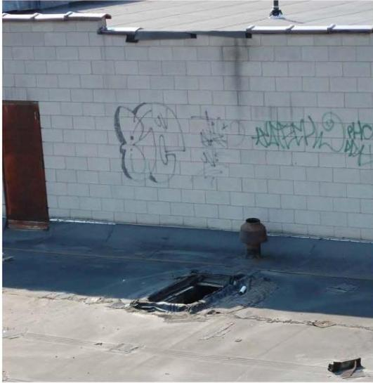
*Photograph 27:* Open roof hatch in the second storey of the original building.
