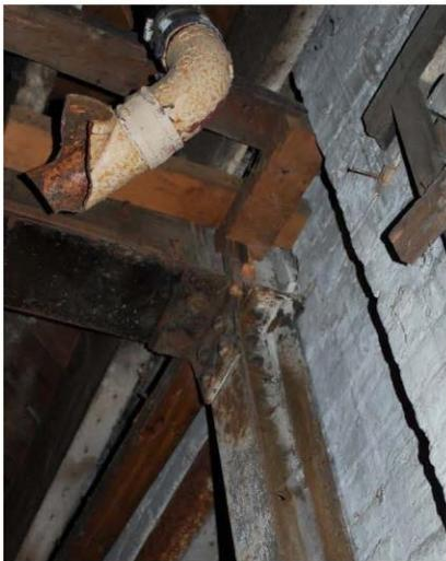
*Photograph 46:* Potential friction connection between the steel and the brick wall.
