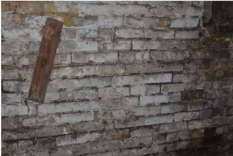
Photo No. 07: Basement Wall with Severe loss of Mortar
