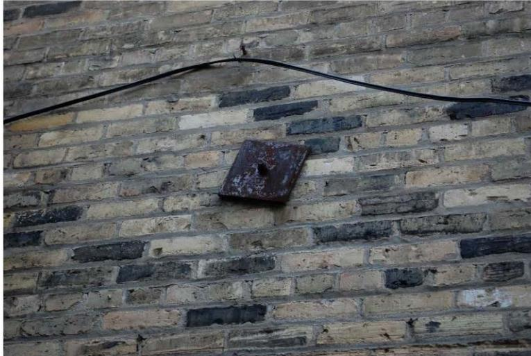
*Photograph 24:* Tie-back plates on the exterior of the middle addition to connect the floor and wall system.
