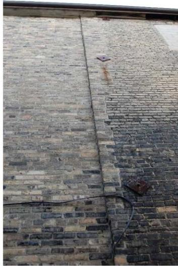
*Photograph 4:* Joint between the two three-storey building sections.
