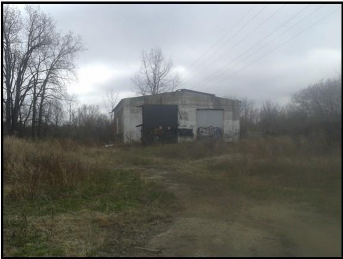
Photo of Subject Property – 529 Philip Street – Dilapidated Former Auto Repair Garage
