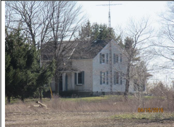
Image 3: View of the house located at 5067 Cook Road.
