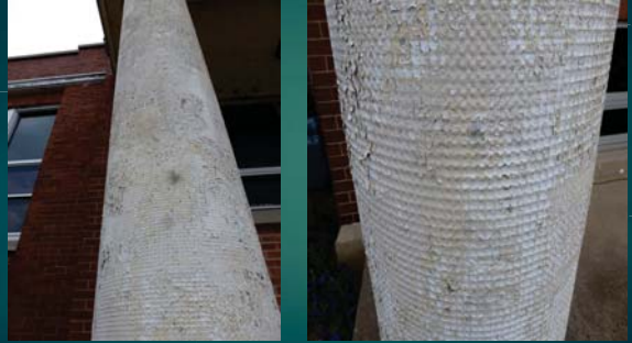
Structural - Front Pillars
