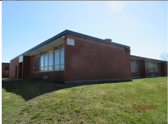
Image 6: 1963 wing of the former school.
