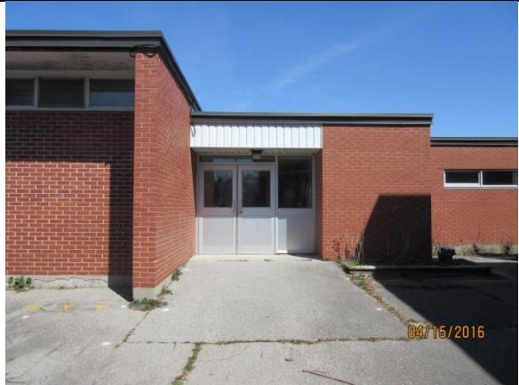
Image 4: 1969 library addition (and main entry).
