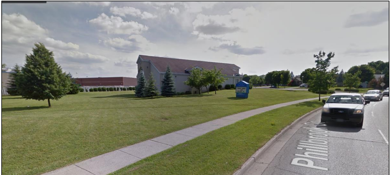
Figure 1: Streetview of existing structure from Phillbrook Dr
