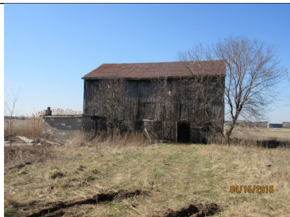
Image 6: Barn located at 5067 Cook Road.
