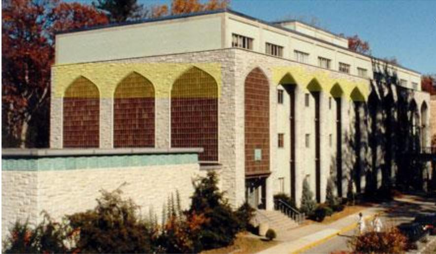
**Buttress:** A buttress is an exterior support projecting from the face of a wall. Walls were often stiffened by external buttresses designed to carry weight of the roof while still allowing walls to be pierced by large windows. An example at Loyola is Jenkins Hall:
