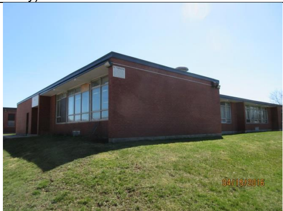
Image 6: 1963 wing of the former school.
