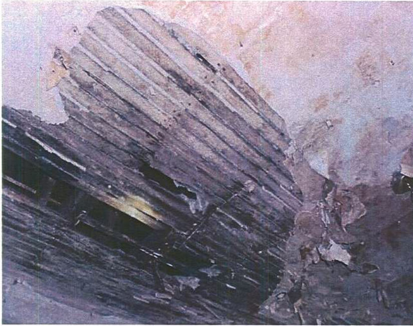
Damage to the upper floor ceiling because of water leakage.
