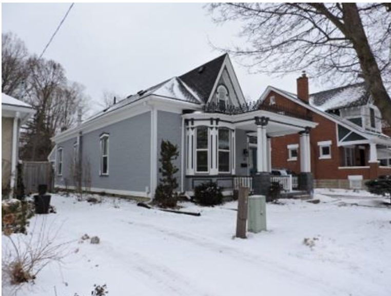
Image 2: West elevation of the building located at 68 Bruce Street (courtesy of Amy Barnes).
