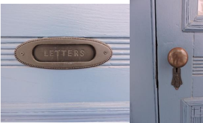
Photo 8: Details of finishing on front door. Letter box opening (left) and metal door knob (right) (AB, 2016)
