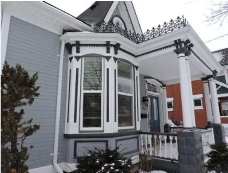
Photo 10: Detail of facade bay window and porch (AB, 2016)
