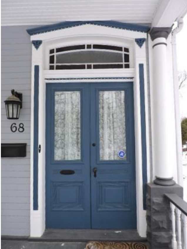
Photo 7: Front entranceway (AB, 2016)
