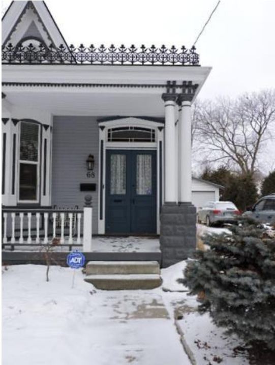
Photo 6: Front entrance and porch (AB, 2016)
