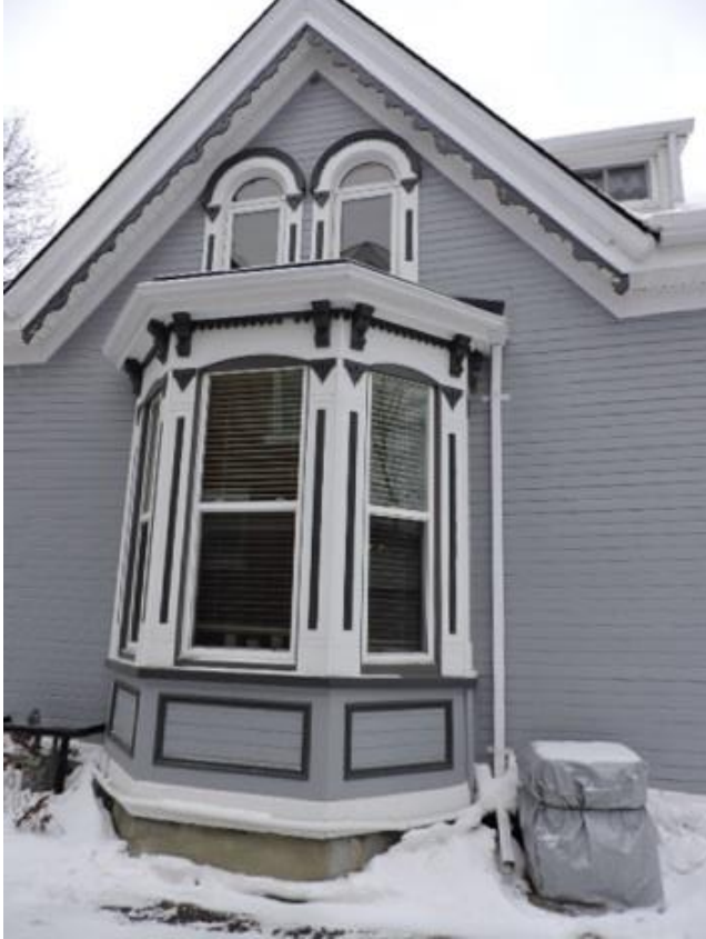
Photo 5: East elevation bay window (AB, 2016)
