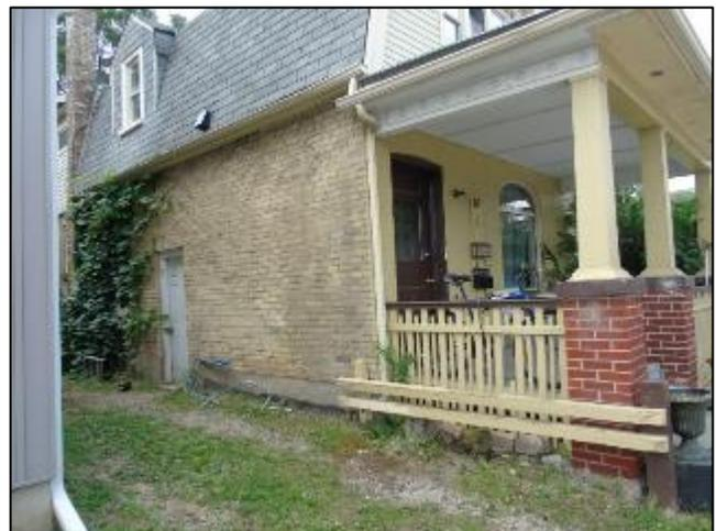
*Plate 26: East facade of 88 Oxford Street West showing side door and brick-work where recessed front entrance may have been*
