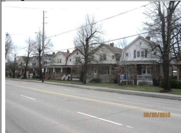
Image 17: 136-146 Wharncliffe Road North (6 properties).
