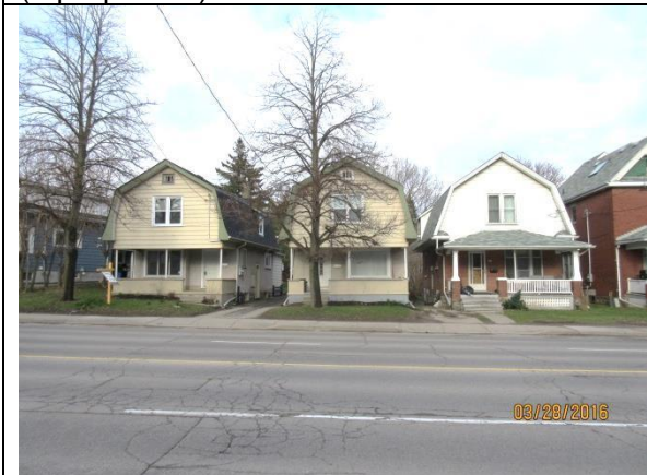
Image 19: 197-201 Wharncliffe Road North (3 properties).
